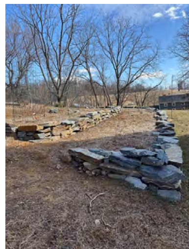
Backyard terraces Photo courtesy of Gaye Mara
